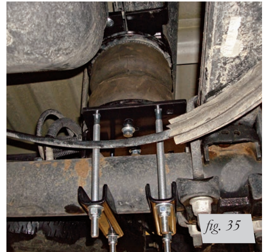
Left side (driver's): front view of installation.
